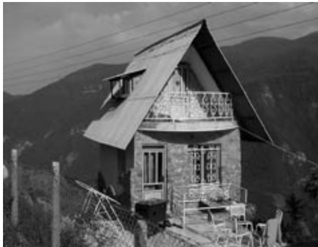
Caretaker's house perched in the mountains of Iran.
